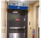
Several factors are taken into consideration when choosing an industrial air curtain, the most important of which are the size of the entrance, the required temperature, humidity, noise requirements, the extent of the required protection from dust and insects, energy efficiency, and the project budget.
